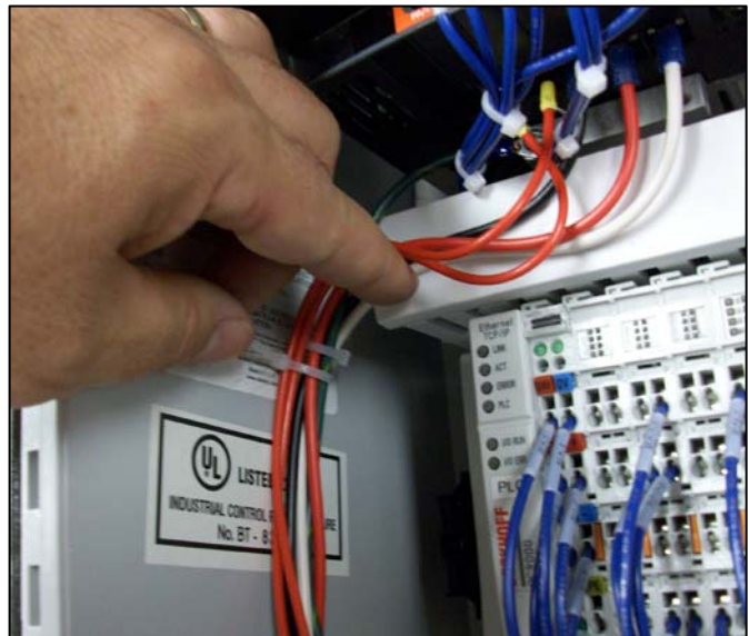
Pic #11: Secure Wires
