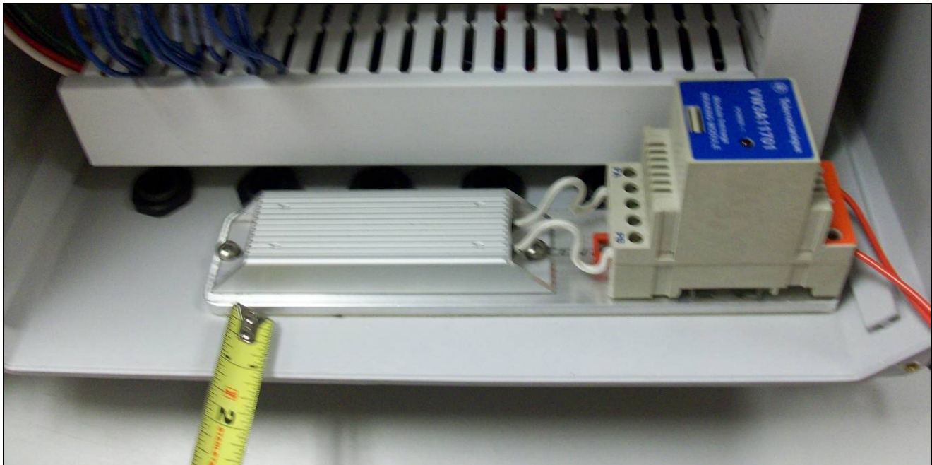
Pic #3: Locate 1" from Edge
