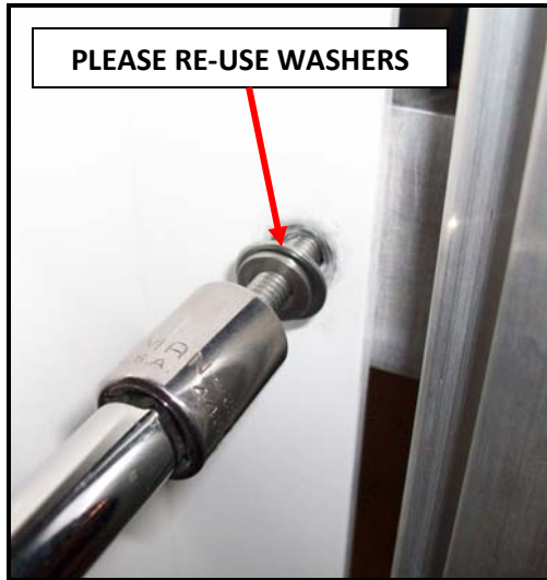
PIC #6: REPLACE EXISTING BOLTS
