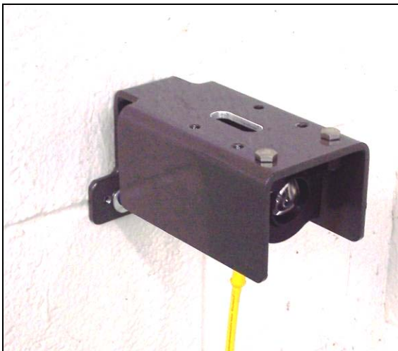
Pic #8: Photo-Eye Guard Wall Mounted
