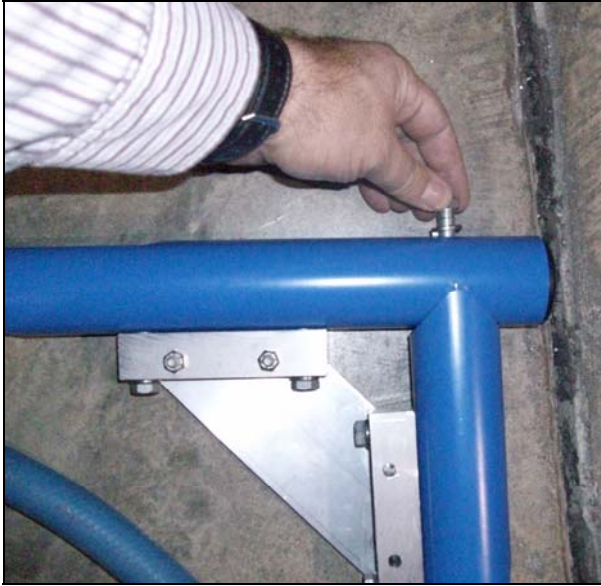
Pic #6: Assembling Passenger Leg
