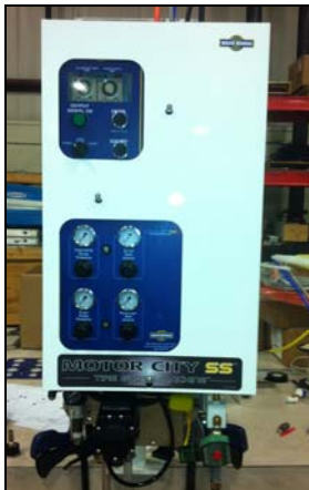
Pic #1: Pumping Station
